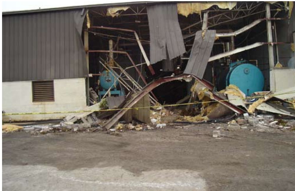
Photo #6 – View of East Wall from Outside Plant
